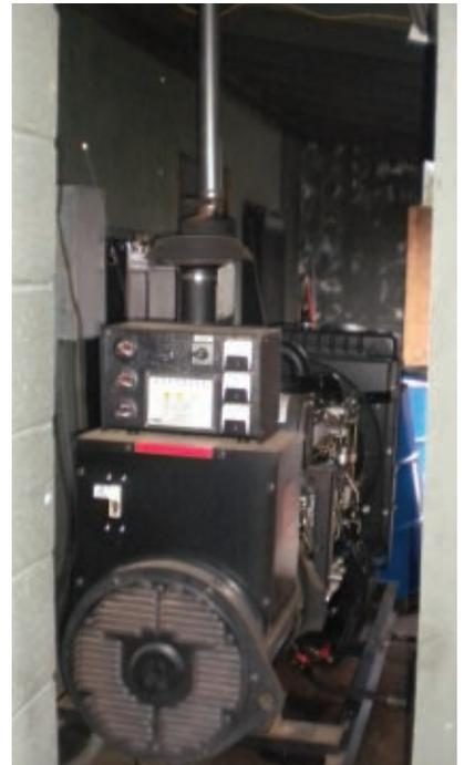
**An existing 60 kW Isuzu-powered generator set has delivered more than 25,000 hours of reliable service at the camp.**
